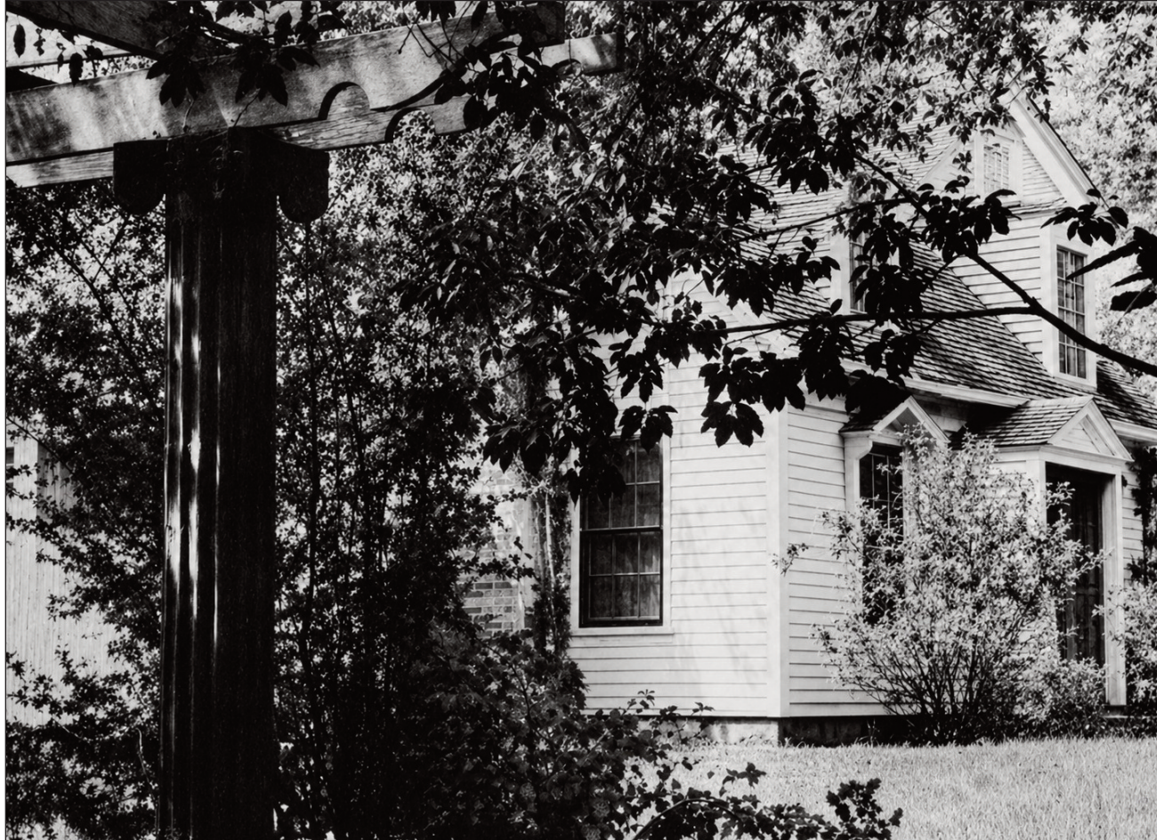
From Illustrated Press of Liberty County, Thursday, July 20, 1967 – The picturesque Humphreys' homes in Liberty are being torn down in Liberty to make way for new construction.
